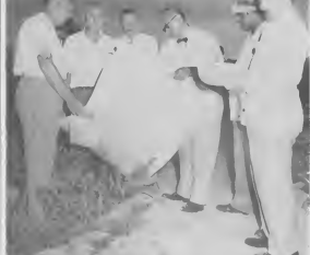
"IT WILL GO right here," says architect Morris Lapidus to a group of Aruba government and businessmen. He was speaking of the new Aruba Caribbean Hotel, which he designed, and which will soon be rising from the sands at Palm Beach.
